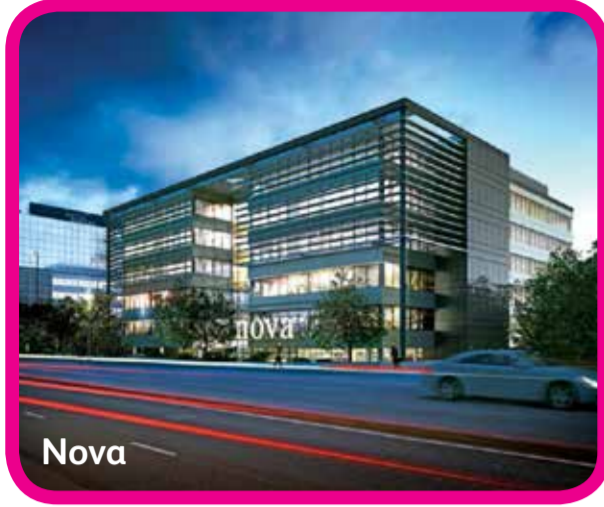
Nova London Road and County Oak Way junction improvements
